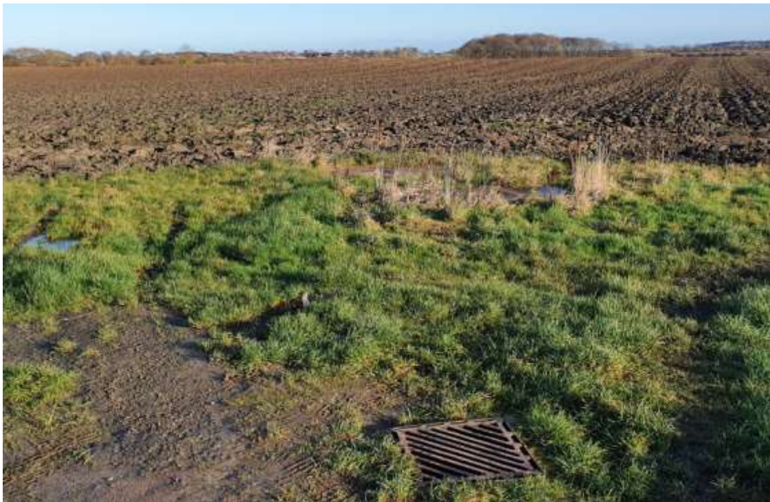
Figure 7: View looking north east from the south west of the main site showing drainage and manholes.
